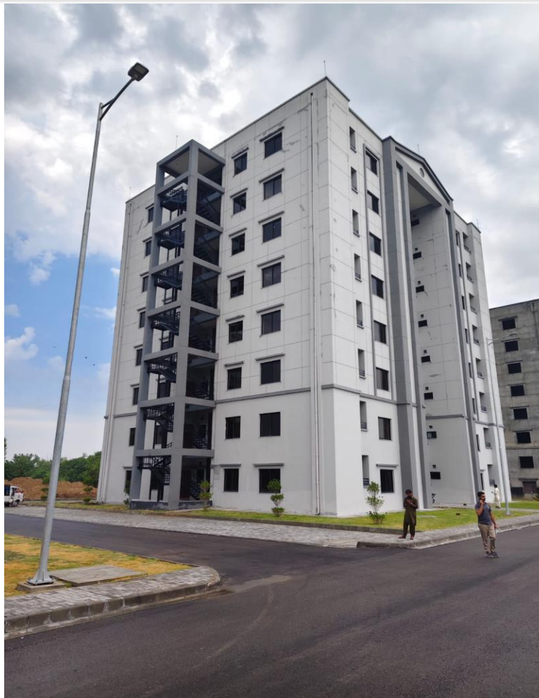
Figure 5. Newly constructed G+7 building at POF Wah Cantt
